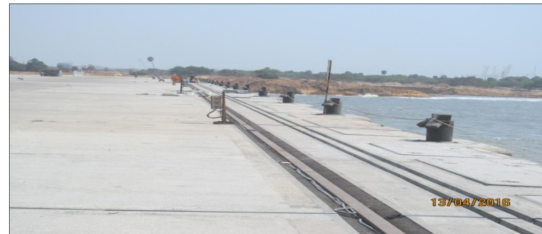
Ennore container terminal, Chennai
