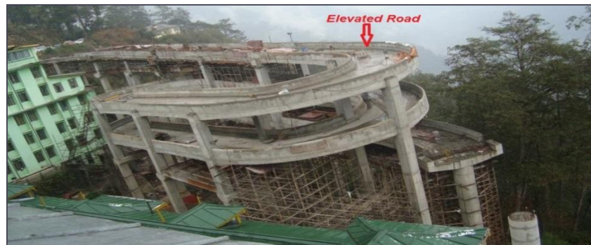
Piling & Civil Arctech, Gangtok
