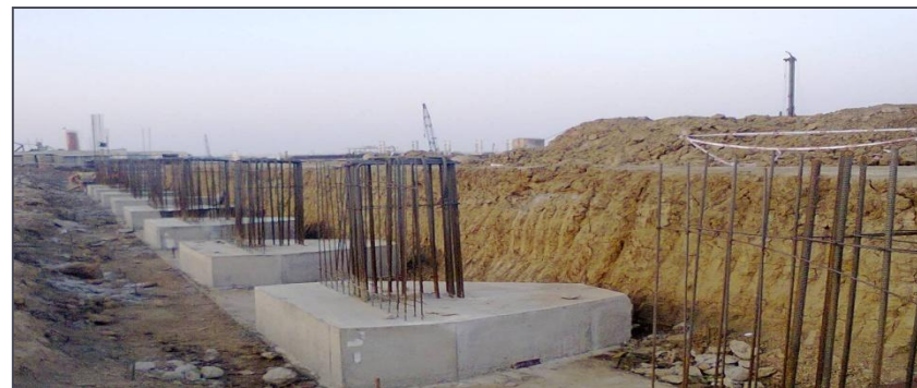
Foundation BASE, Dahej
