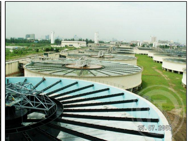
Bang Khen Water Treatment Plant , Bangkok
