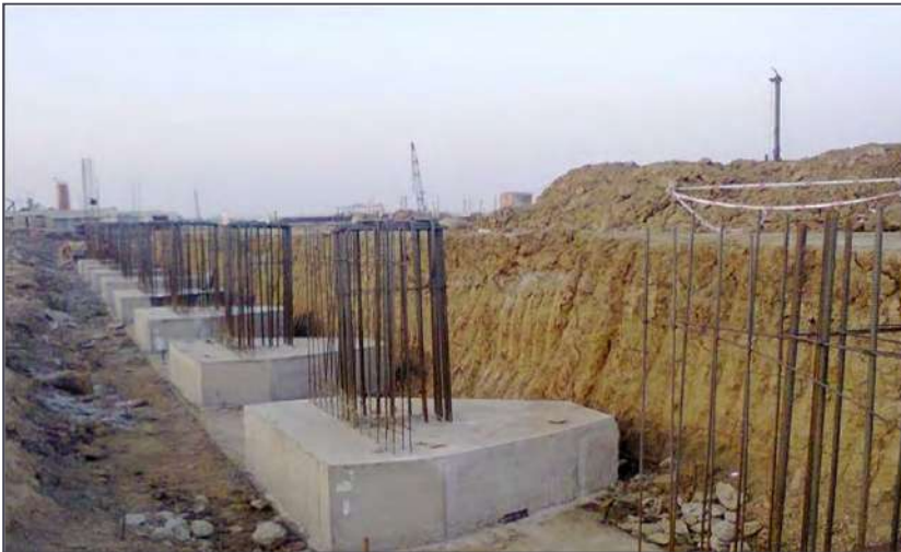
Foundation BASF, Dahej
