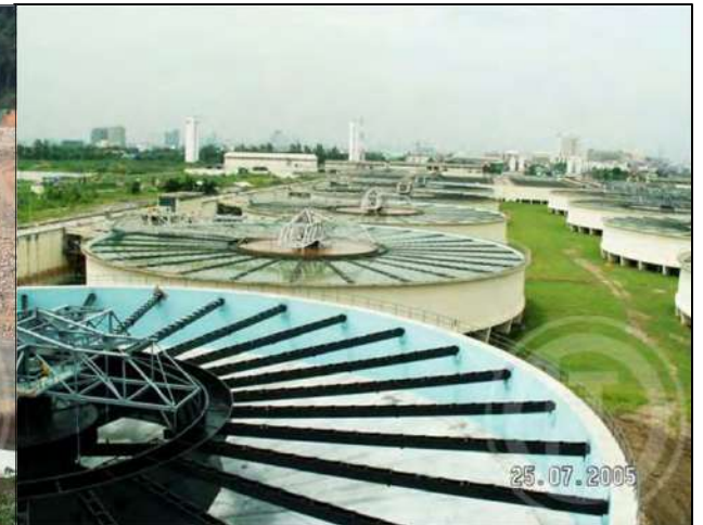
Bang Khen Water Treatment Plant , Bangkok
