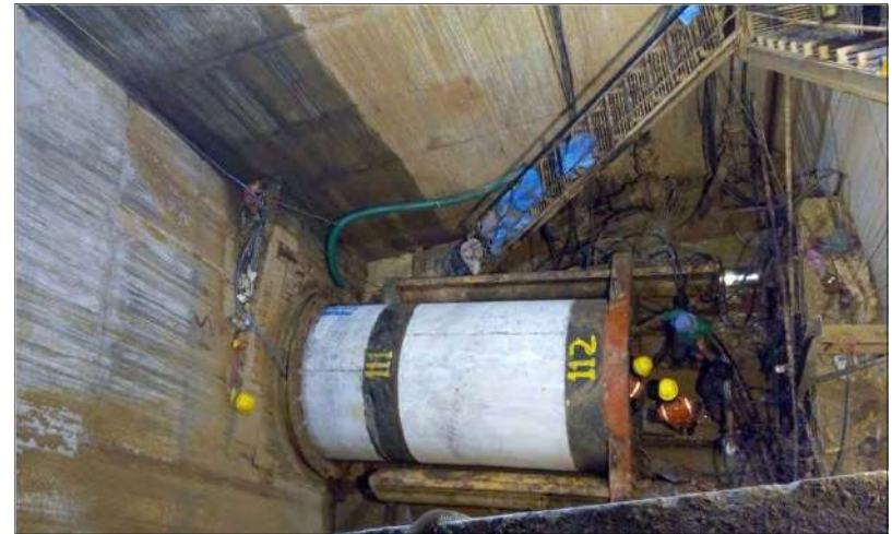
VMSS – Micro Tunneling Vadodara
