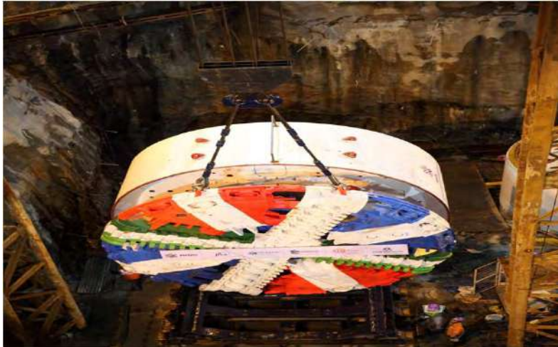
Lowering of TBM, Mumbai Metro L3
