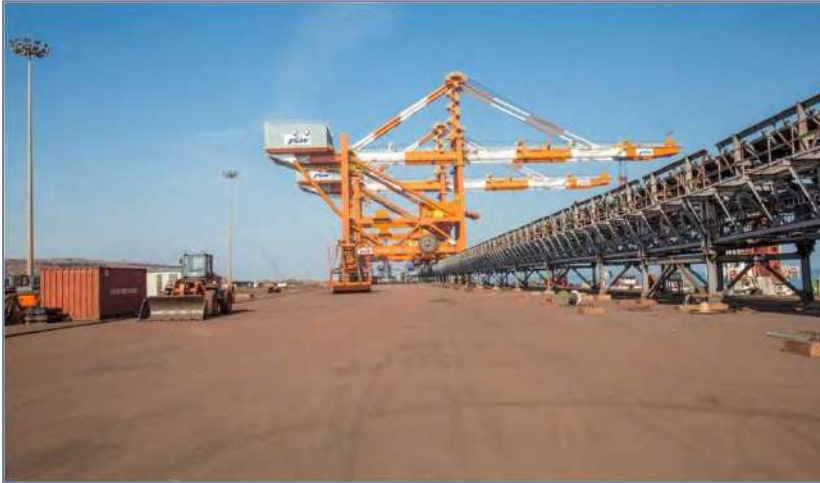
Piling & Civil Works for JSW, Jaigad
