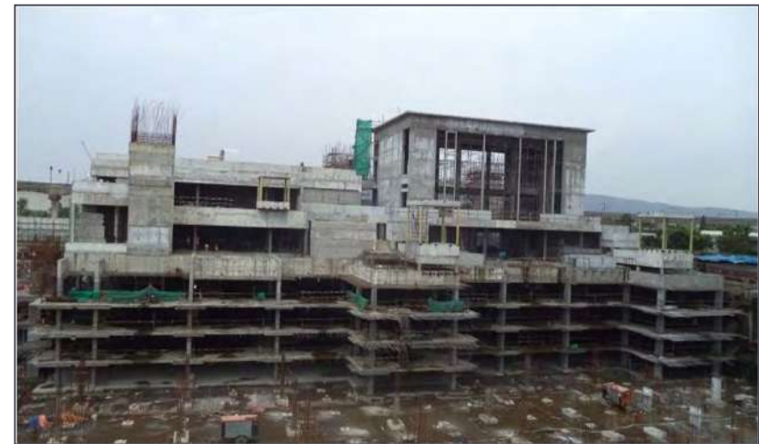
Civil Works Wadala
