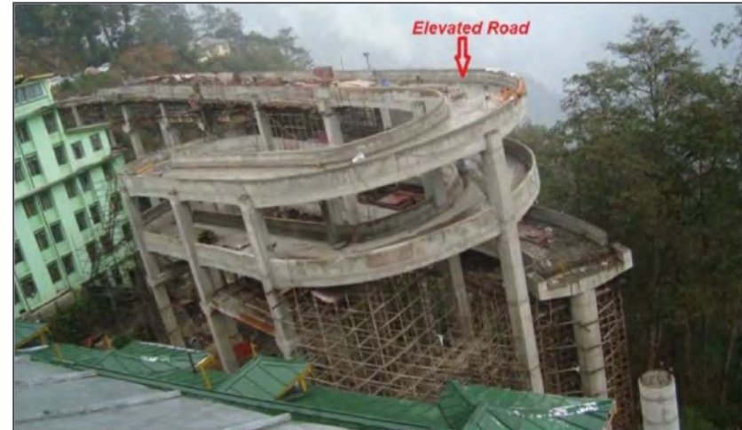
Piling & Civil Arctech, Gangtok
