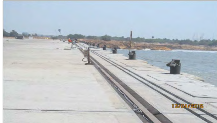
Ennore Container Terminal, Chennai
