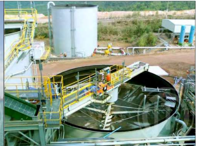
HDPE Tailing and Decant Piping Installation
