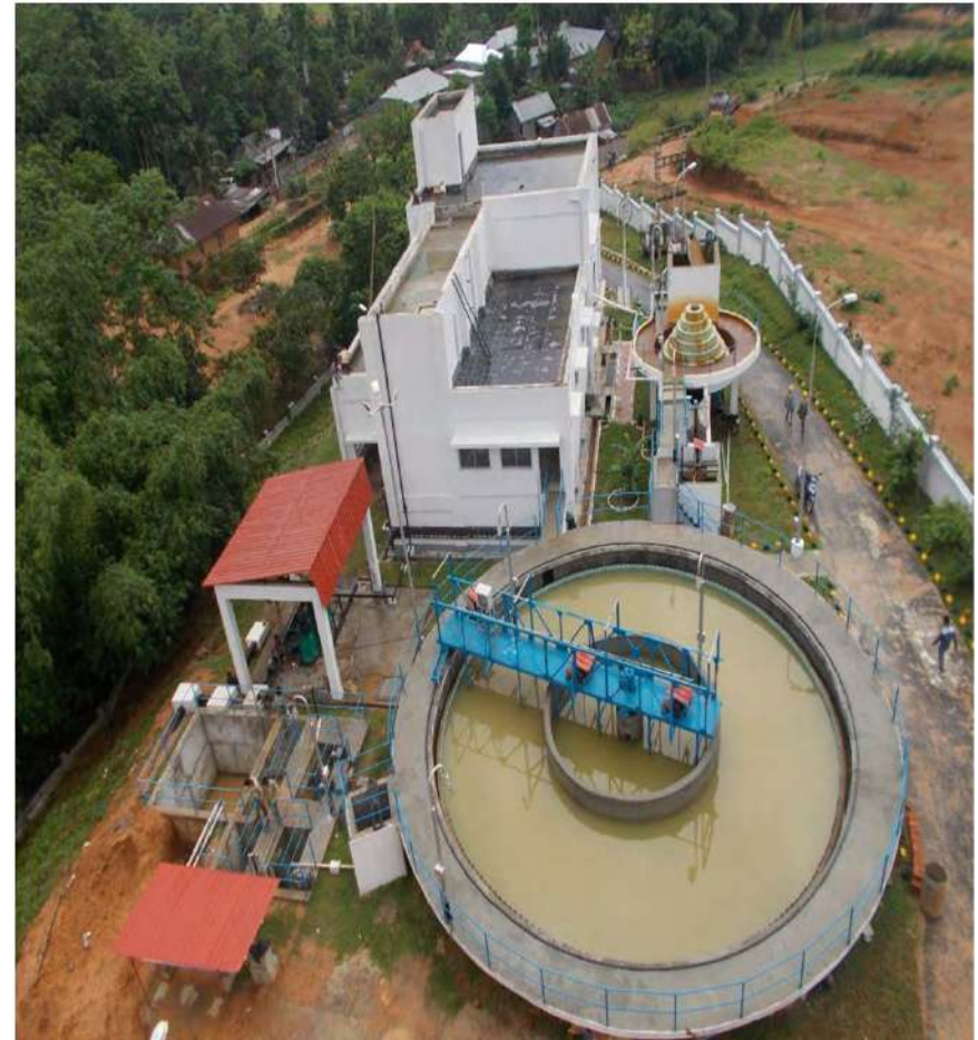
Agartala WTP project
