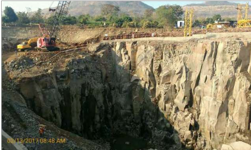
Bhama Ashed Water Supply Project
