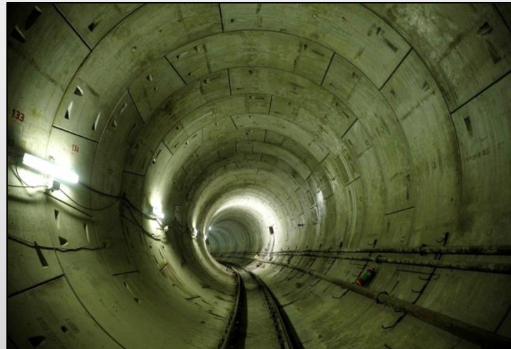
TBM Tunnel, Mumbai
