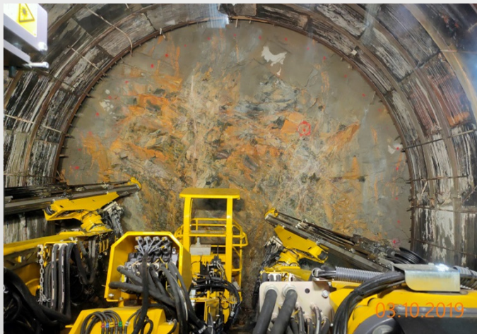
Drill & Blast Tunnel for Indian Railways
