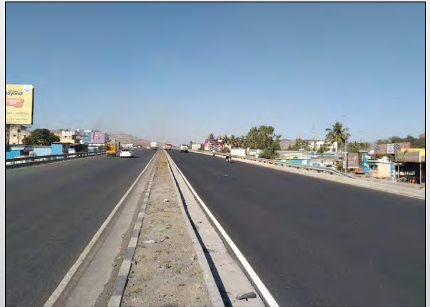
Pune Satara Road Project
