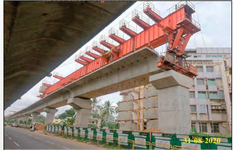
Bangalore Elevated Metro Project
