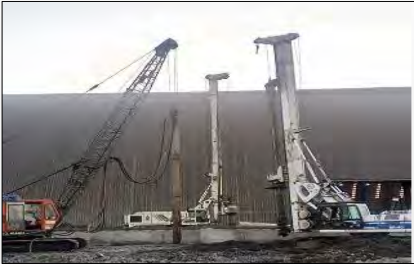
Stone Column Project, Maharashtra
