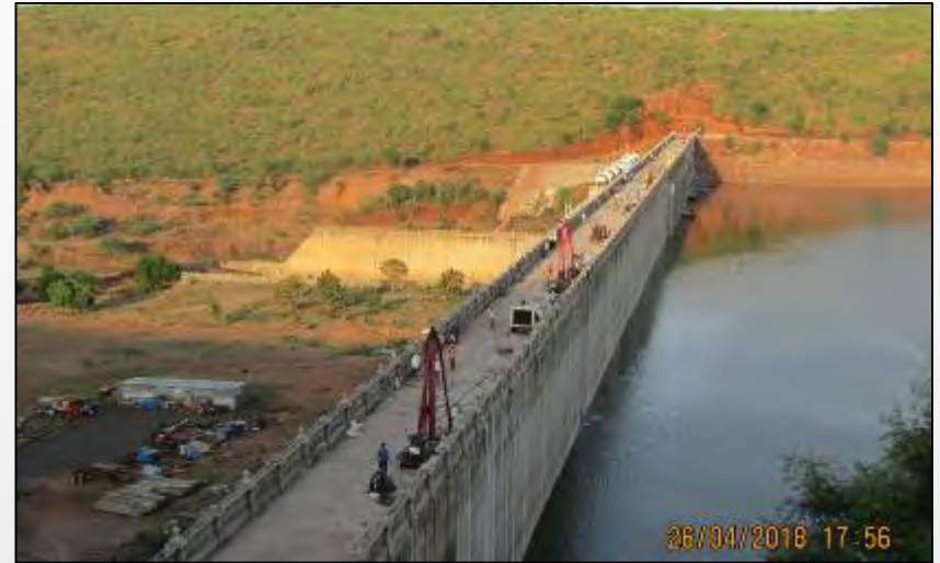
Rehabilitation of Markandeya Dam, Karnataka
