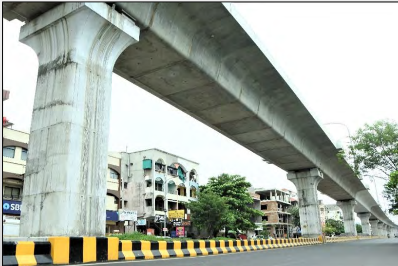
Nagpur Metro Elevated Project
