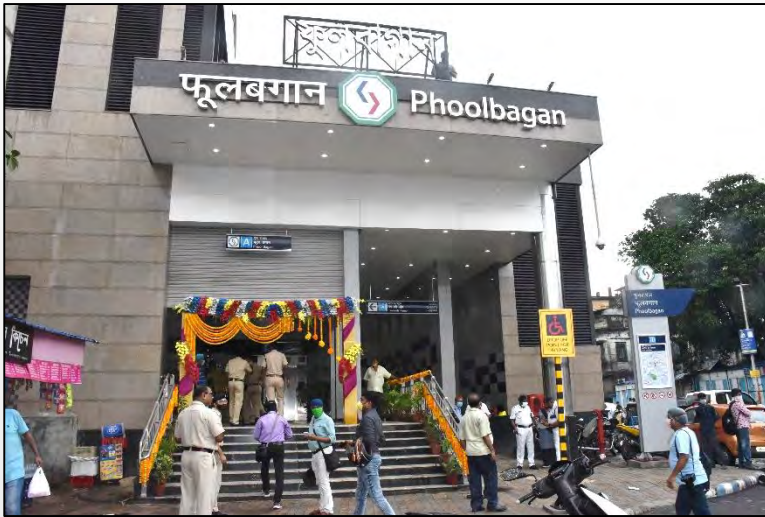
Phoolbagan Under Ground Metro Station, Kolkata
