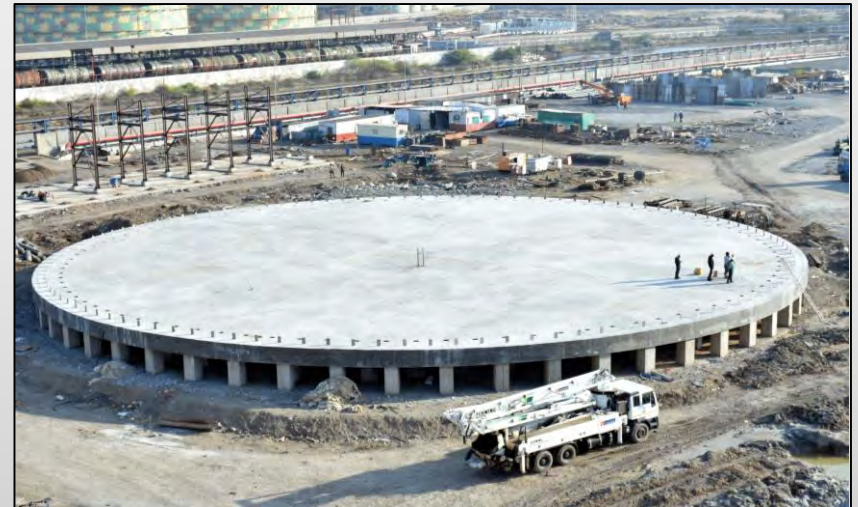
Precast Piling Project, Kandla
