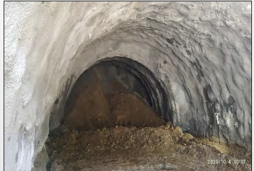
Railway Tunnel Project, Sikkim
