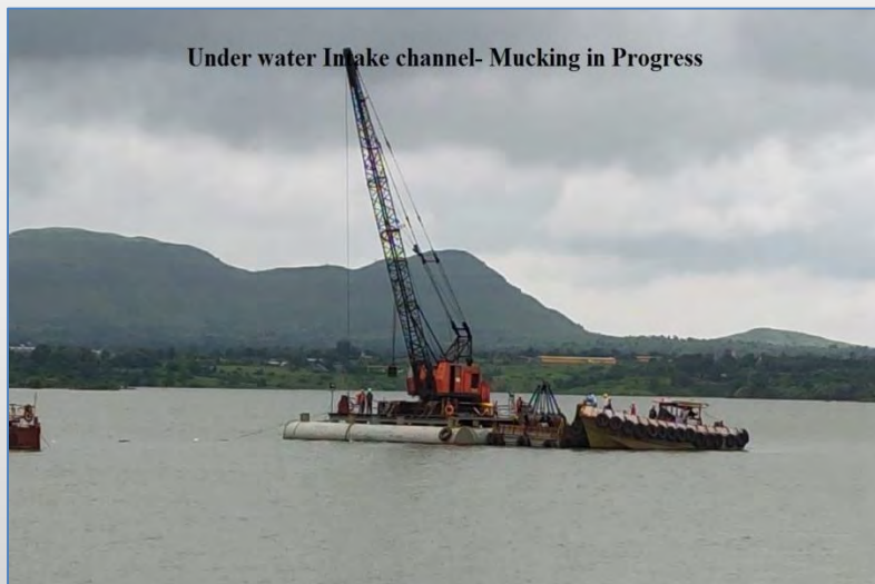
Irrigation Project, Bhama, Pune
