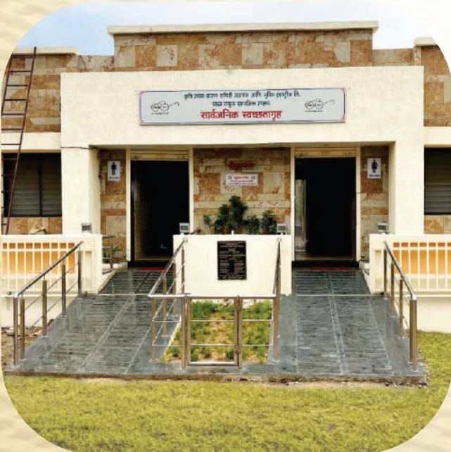
APMC Toilet Block, Jalgaon (Maharashtra)
