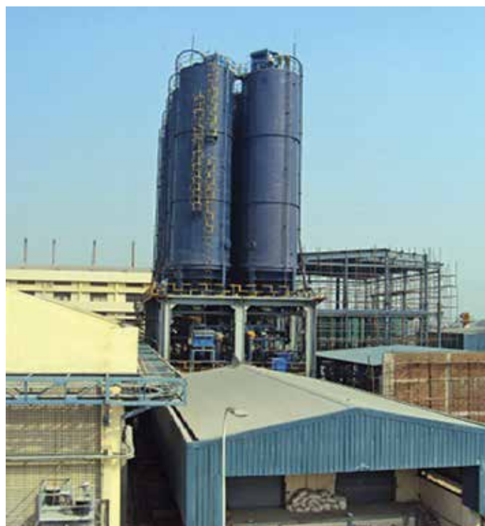
Silo System at Jainpur
