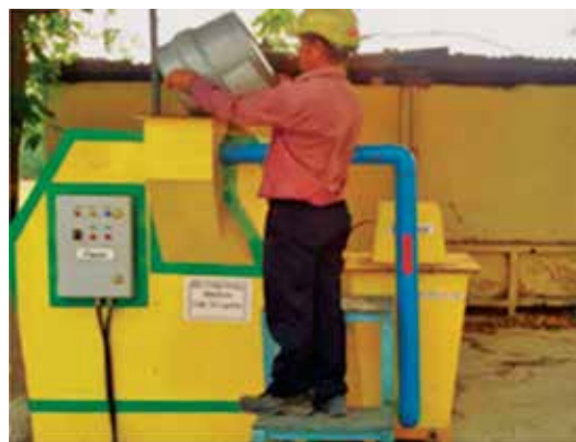
Biocompost Machine (Organic Waste to Fertilizer) at Bawal Plant
