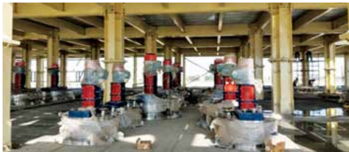
OEM mixers installed at Saykha Plant
