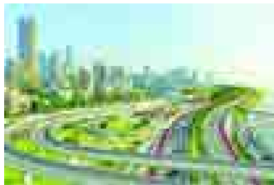
Mumbai Coastal Road (Mumbai, MH)
