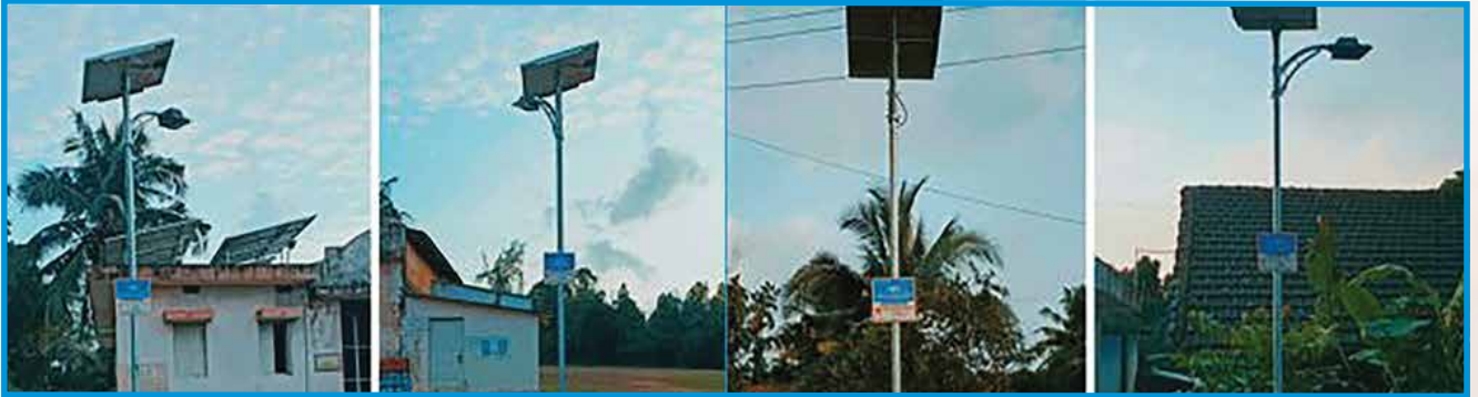
▲ Solar street lights installed
