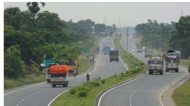
Km 341 (Farakka Raiganj Highway)
