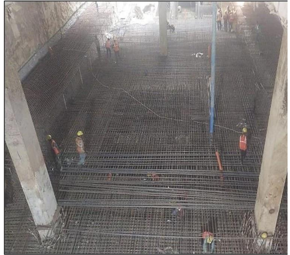
Station Base slab works Grid 5-8
