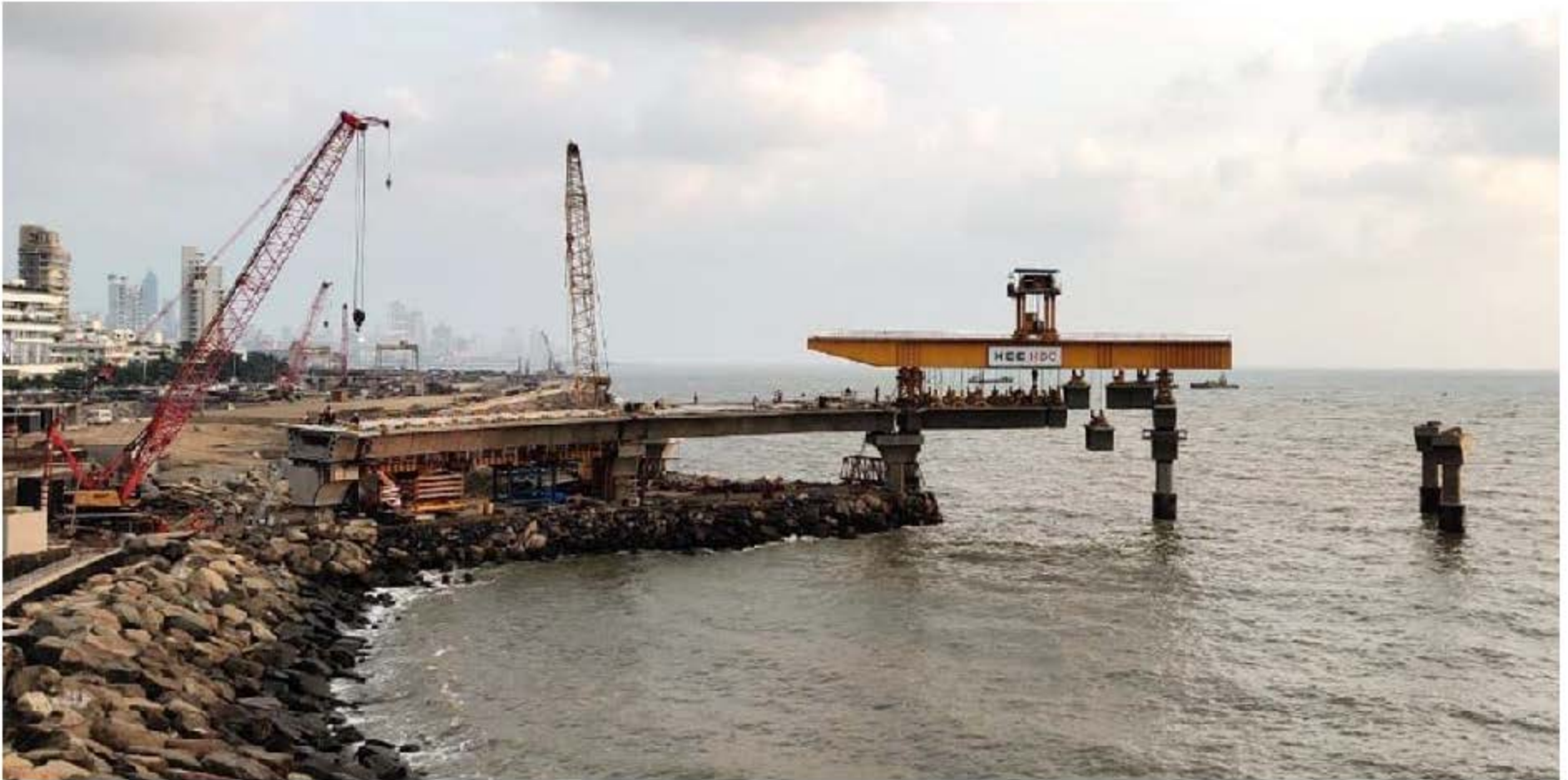
Arm – 2 Segment Launching
