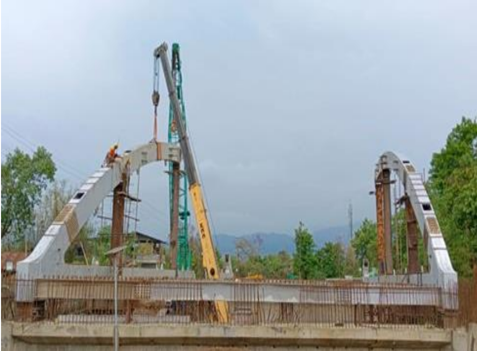
Bow string girder erection @ Bridge 5+411
