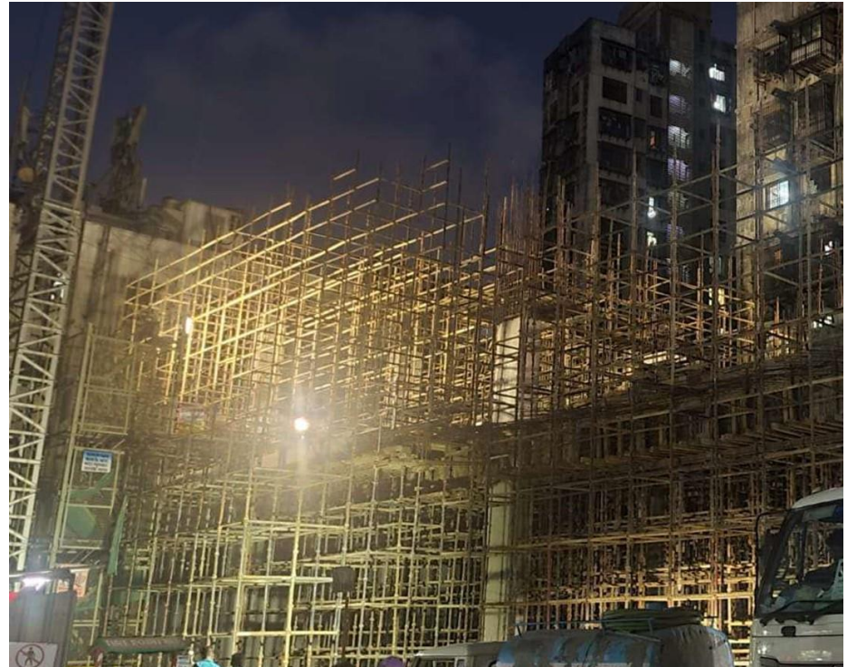
Ancillary Building works
