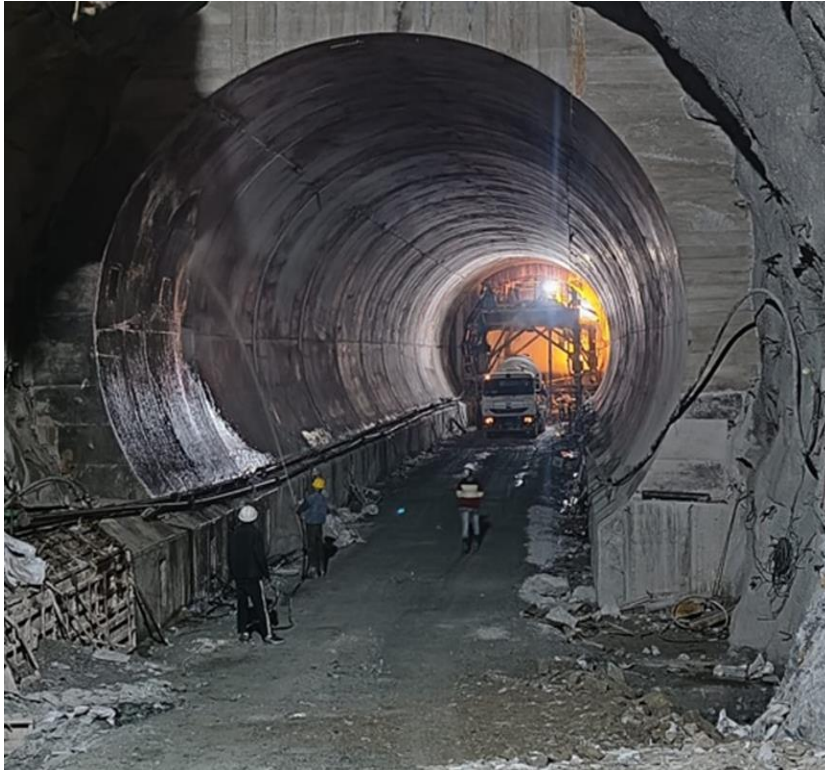
HRT Overt lining
