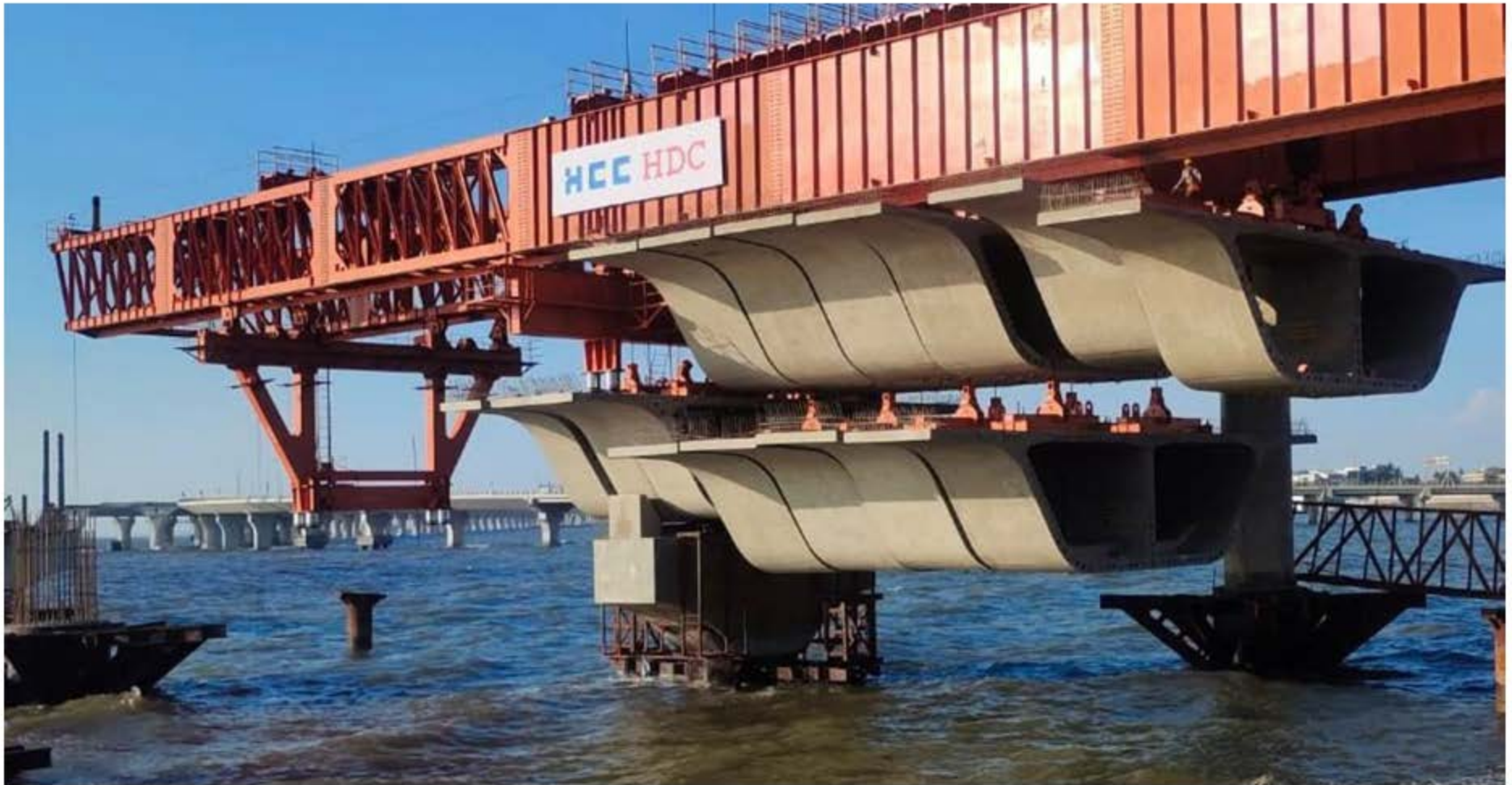
Main Bridge - Segment Launching
