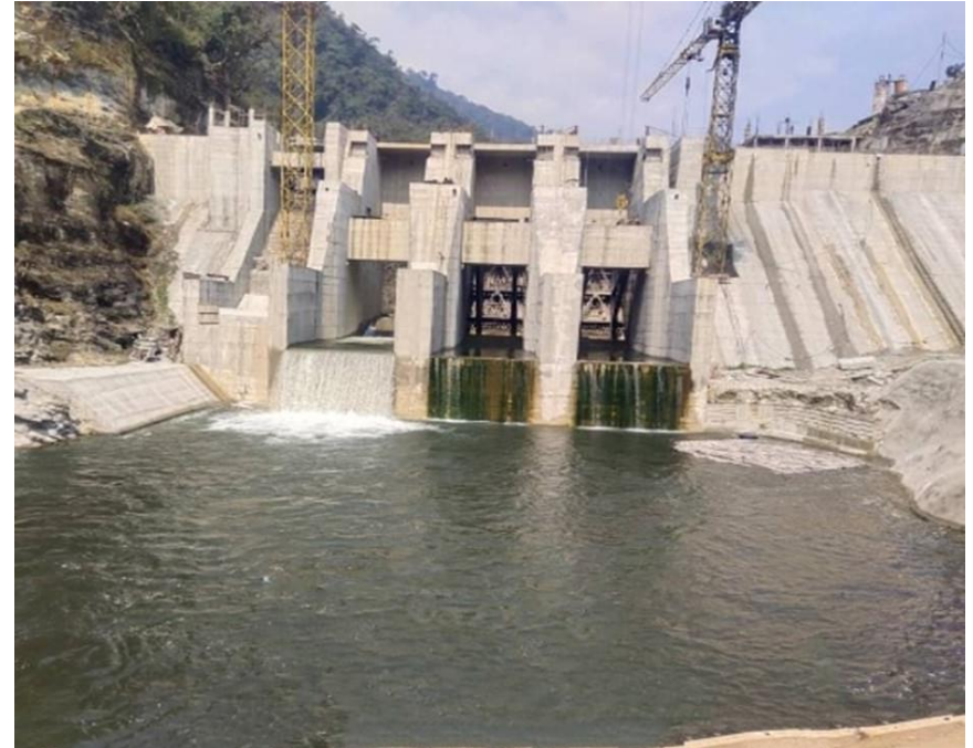
Dam works – River diverted through Radial gates
