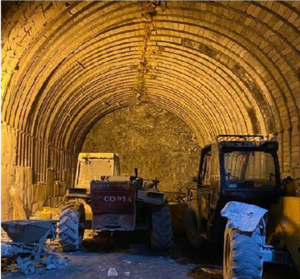
Horizontal Penstock Excavation
