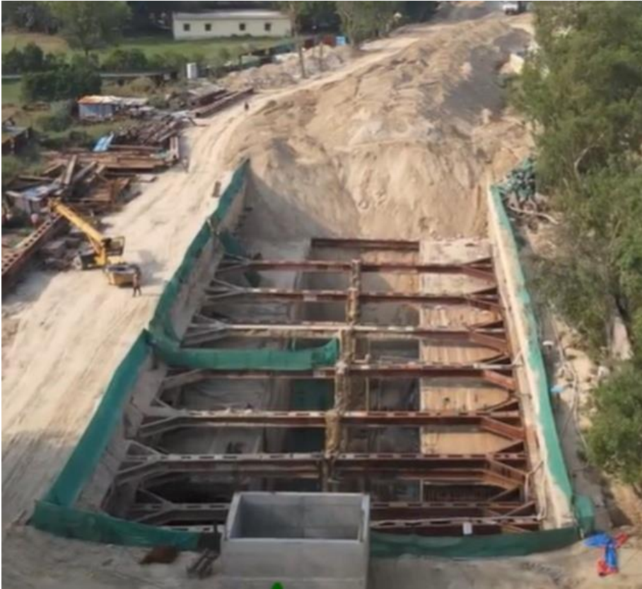
Cut & Cover Roof slab
