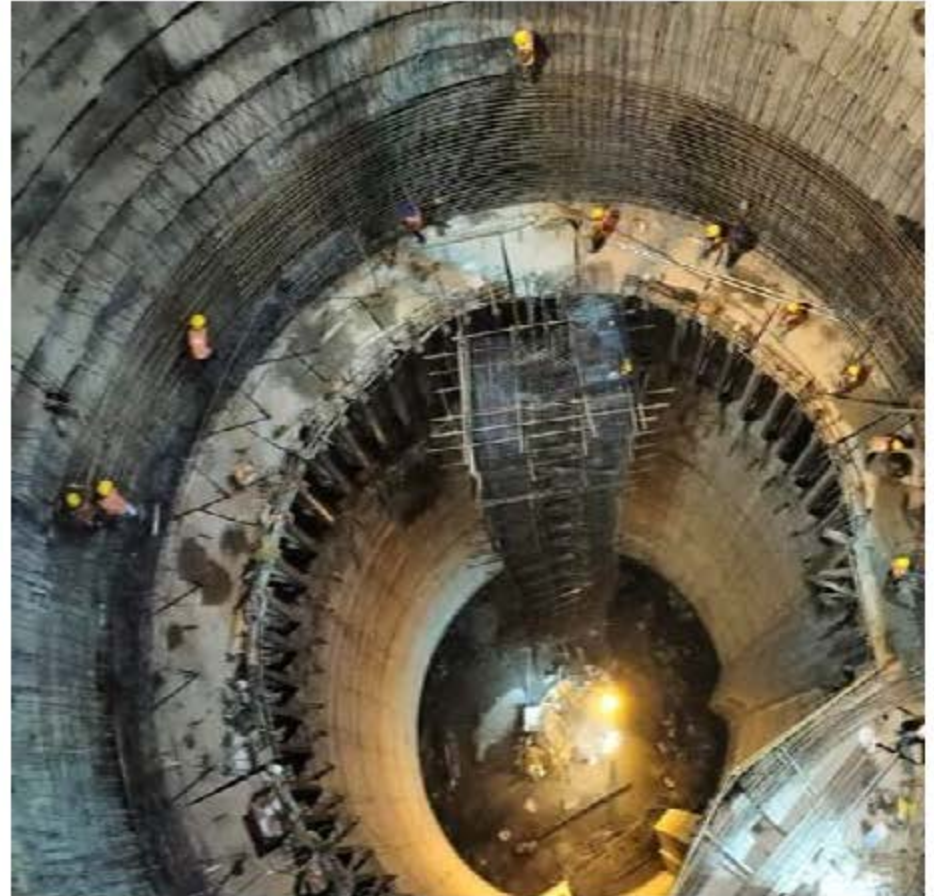
Downstream Surge Shaft Lining
