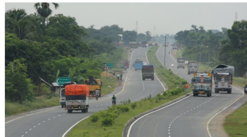
Km 341 (Farakka Raiganj Highway)
