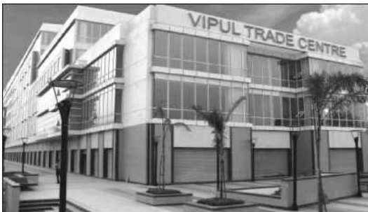
VIPUL TRADE CENTRE, GURGAON
