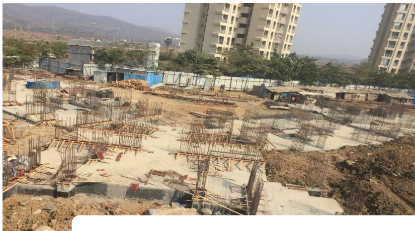
Excavation nearing completion for all 7 towers and Plinth completed for Tower 1,3 & 5
