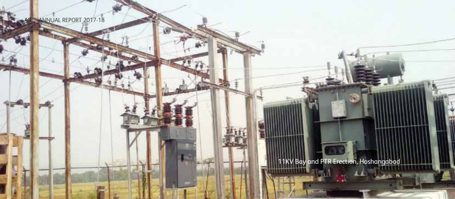
Erection of 33/11 KVA, 5 MA Power transformer, Hoshangabad
