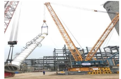
UREA REACTOR TANK INSTALLATION AT RAMAGAUNDAM, TELANGANA
