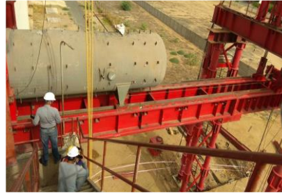
HP HEATER REPLACEMENT 800MW ,CGPL MUNDRA2
