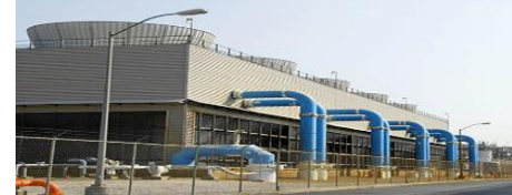
Infrastructure Construction (Civil)
