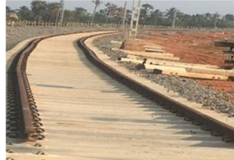
GDV-MTM 37 ,DOUBLING & ELECTRIFICATION WORKS , RVNL
