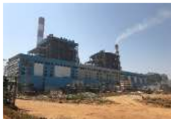
2X660 MW IBTPS, STRUCTURE & STG, BANHARPALLI, BHEL
