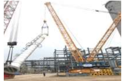
UREA REACTOR TANK INSTALLATION AT RAMAGAUNDAM, TELANGANA
