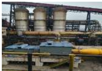
BLAST FURNACE, STEEL PLANT WORK, JSPL, ANGUL
