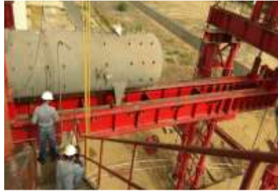
HP HEATER REPLACEMENT 800MW ,CGPL MUNDRA2
