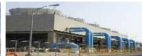
Infrastructure Construction (Civil)
