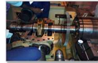
228MW, STEAMTURBINE,SABIYA, KUWAIT, MAIN OIL PUMP OVERHAULING
