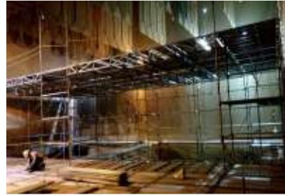
CUPLOCK SCAFFOLDING ERECTION 800MW,MUNDRA
