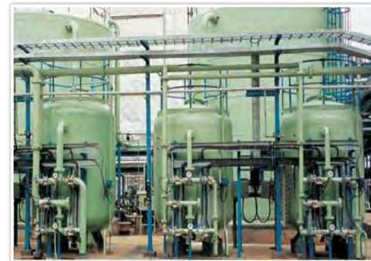
Demineralization Plant for thermal power station
