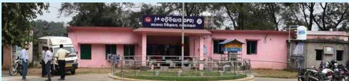
Before Renovation of Primary Health Centre
