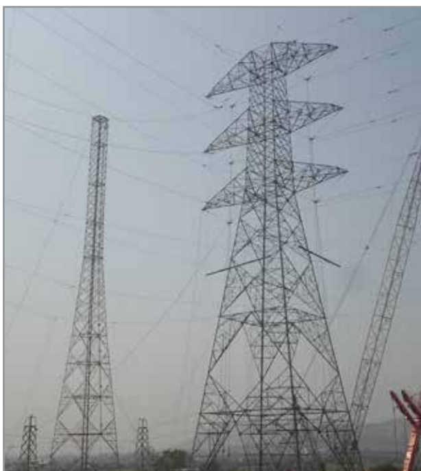
SAM 8550:- 400kV D/C "4DSR (0°-2°)" tower tested for end client- GCCIA and Consultant - Energoprojekt ENTEL
