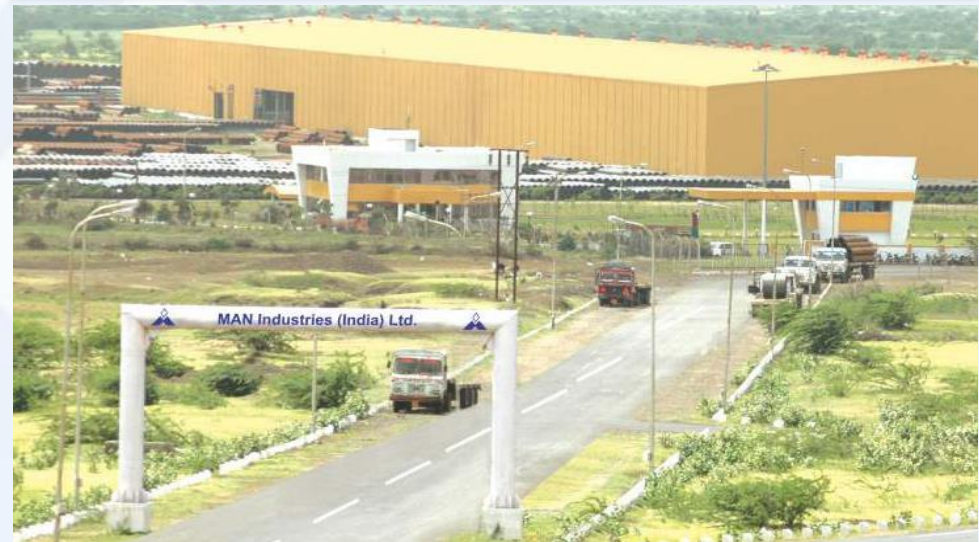
Anjar Plant, Gujarat.
