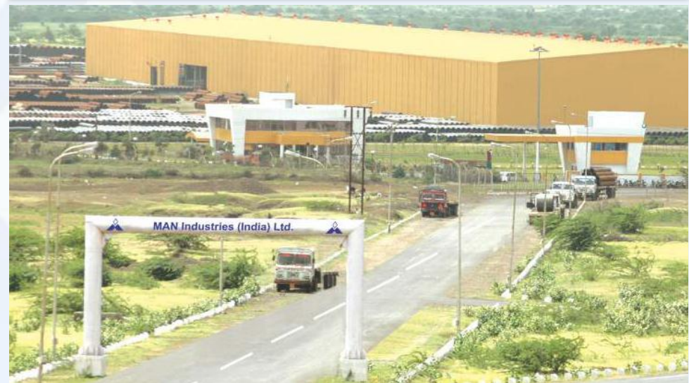
Anjar Plant, Gujarat.
