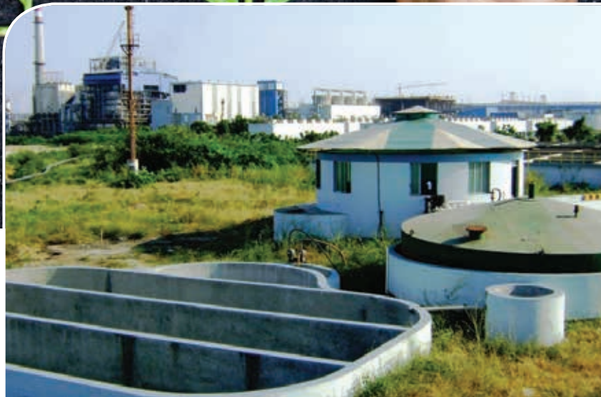
Biogas Plant at Anjar
