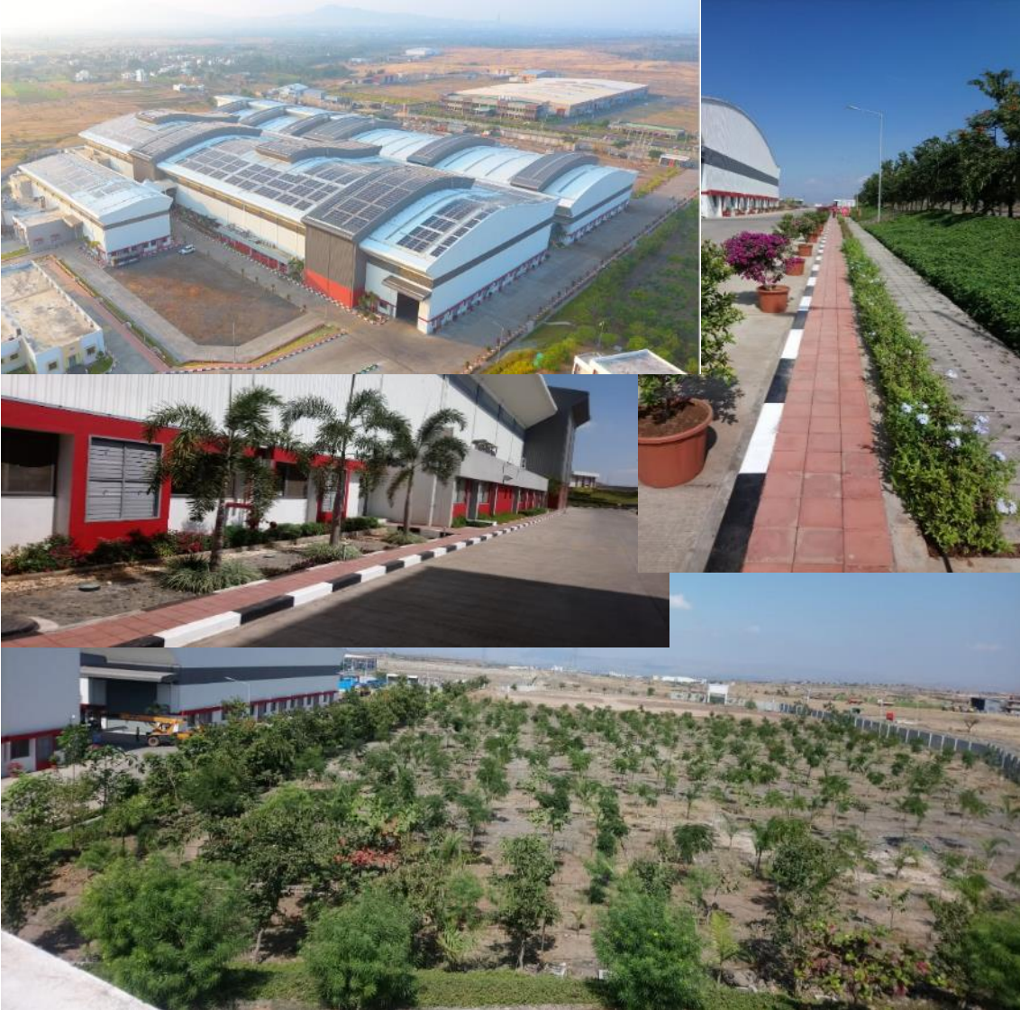
Green Factory: Shirwal Plant
