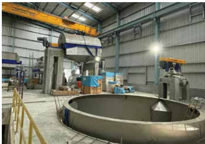
400TPD RCP pulpmill under installation
