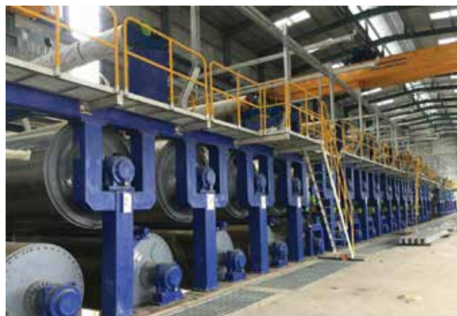
A view of paper machine under installation
