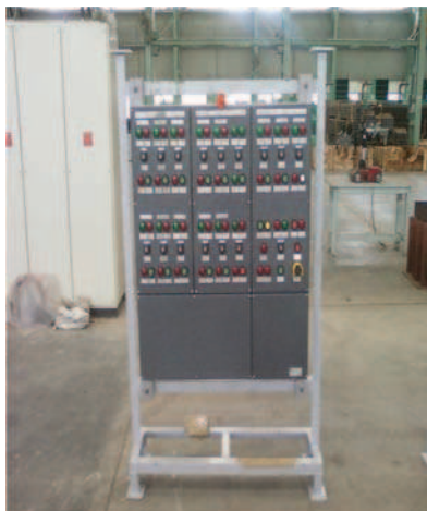
Photo of Relay Based Logic
