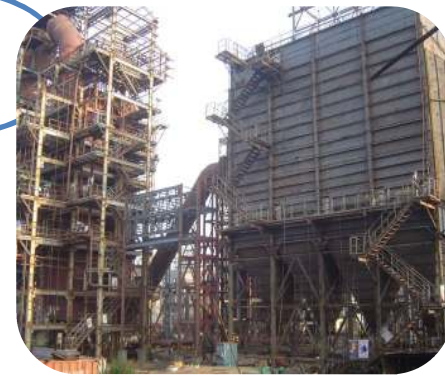
30 MW CPP with DRI
