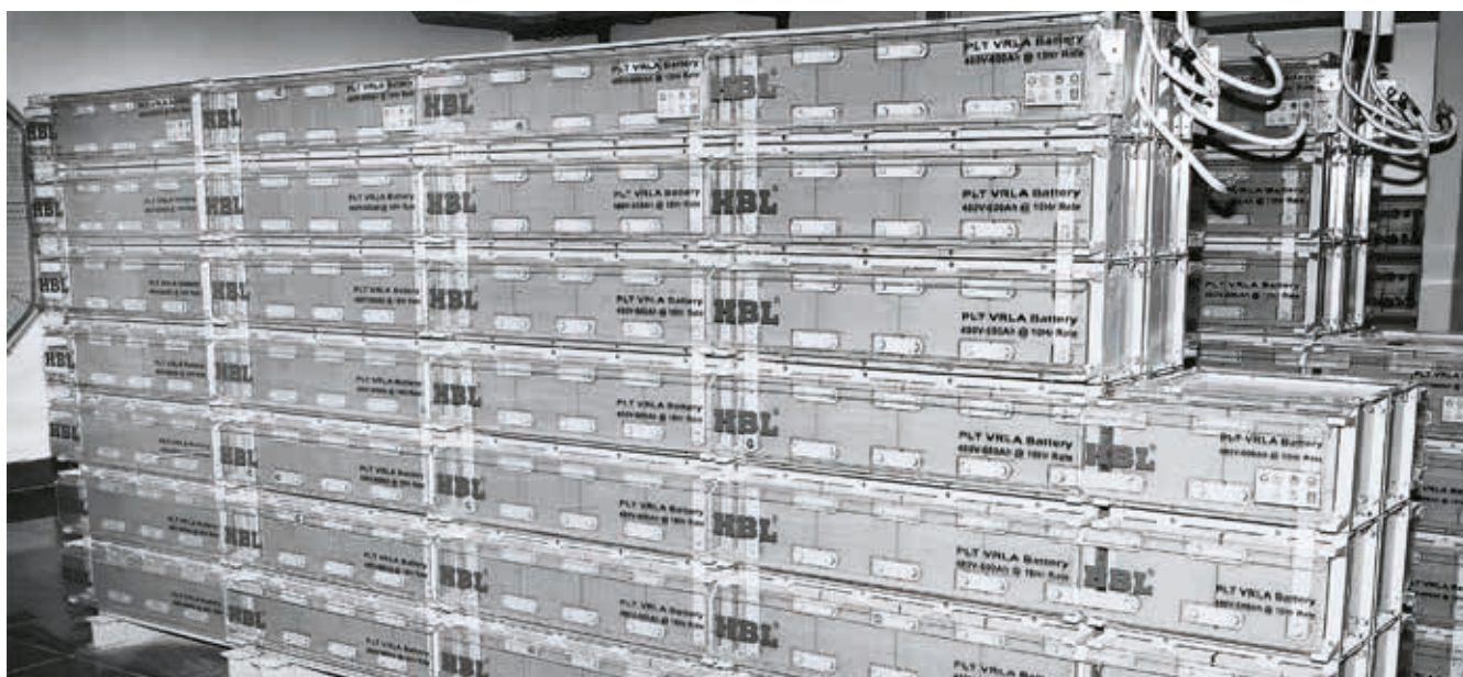
480V-600Ah PLT-VRLA battery installation
