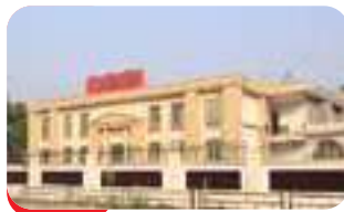
Sahibabad, Uttar Pradesh Switchgears
