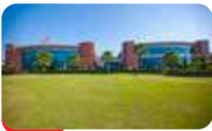
Baddi, Himachal Pradesh Switches and MCB
