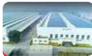
Neemrana, Rajasthan Lighting, Motor, Water Heater
