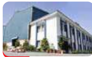
Alwar, Rajasthan Cables
