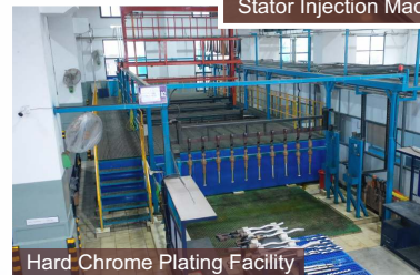
Hard Chrome Plating Facility
