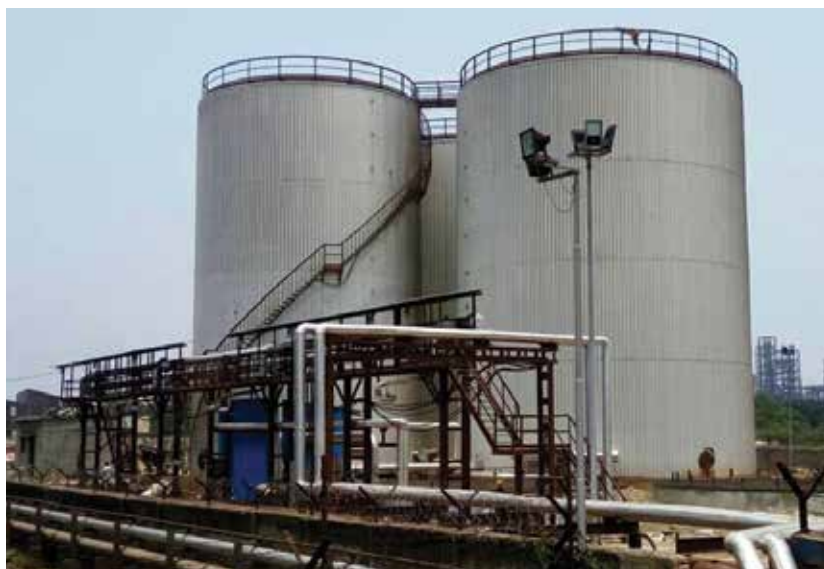
Heated bitumen tanks at Haldia Terminal
