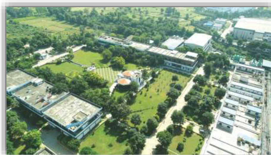
Baddi API Plant: Arial View
