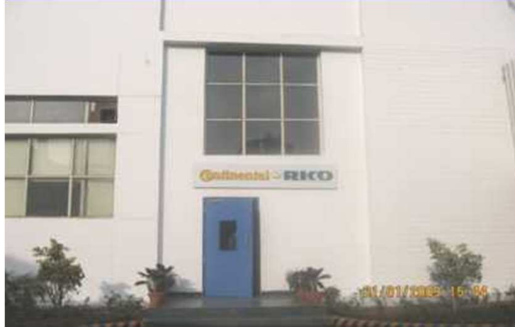
CONTINENTAL RICO (JV) – Gurgaon Hydraulic Brake System
