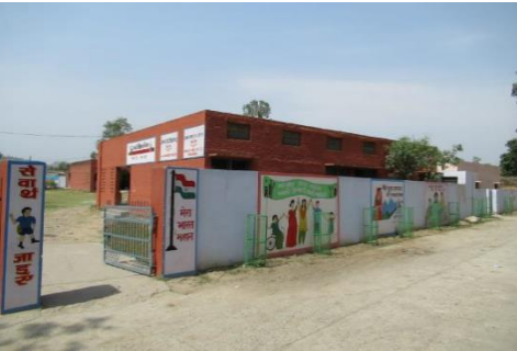
Renovation of Govt. Middle School
