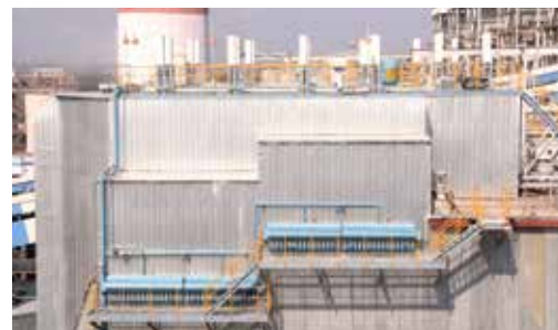
Hybridisation of all ESP's with bag filters, Vedanta Limited – Jharsuguda
