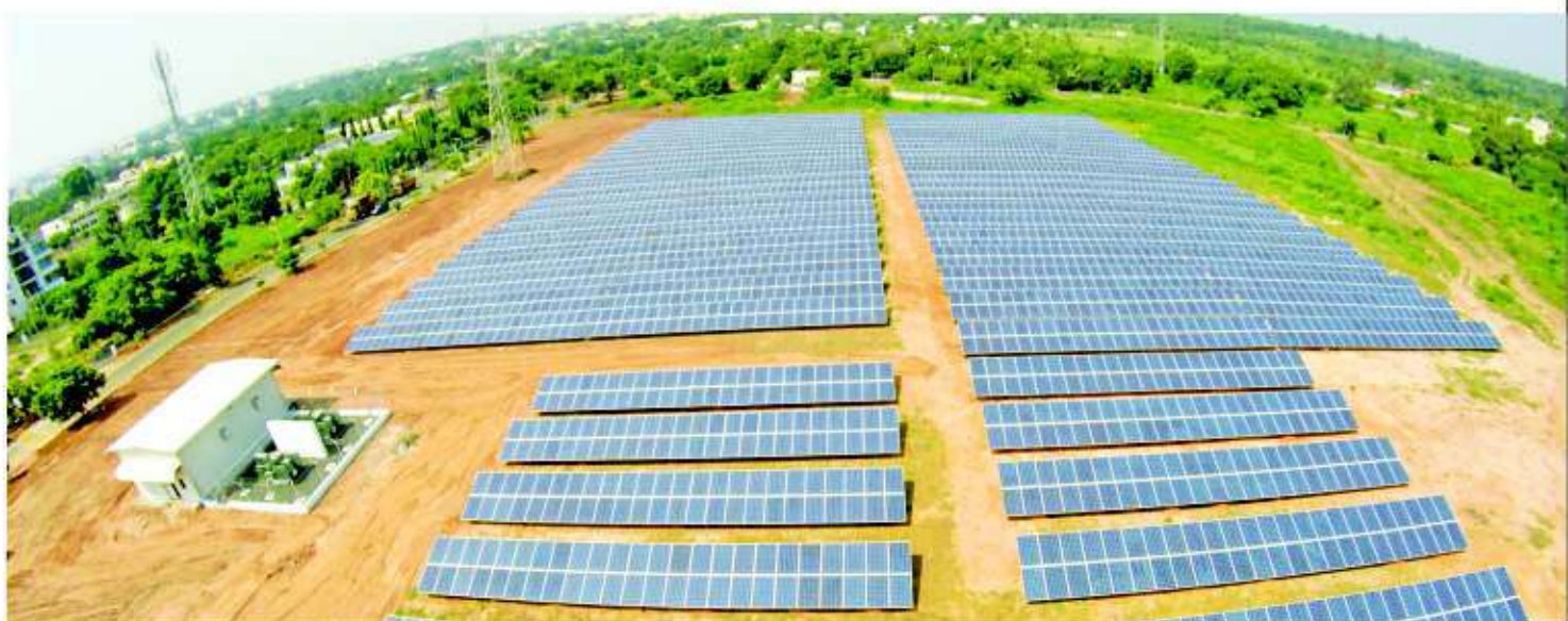
Capturing Energy: 1MW Solar Power Plant, first of its kind at Rajahmundry Base Office Complex in Andhra Pradesh; built in an area of 4.5 acre land costing ₹ 7 crore and envisaged to generate 1.5 million units per annum
