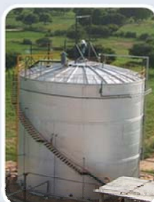
Water and Wastewater Treatment
