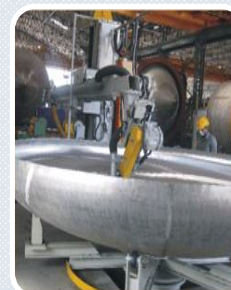
Critical Process Equipment & Systems
