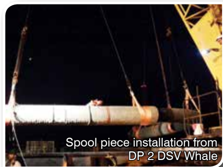
Spool piece installation from DP 2 DSV Whale
