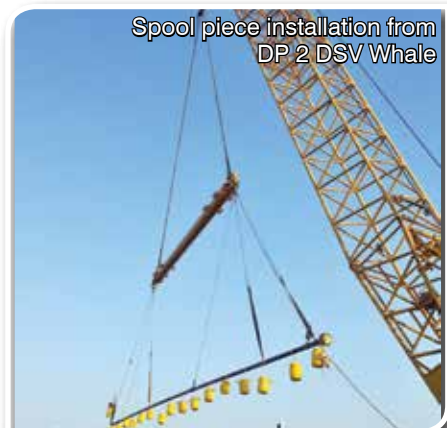
Spool piece installation from DP 2 DSV Whale
