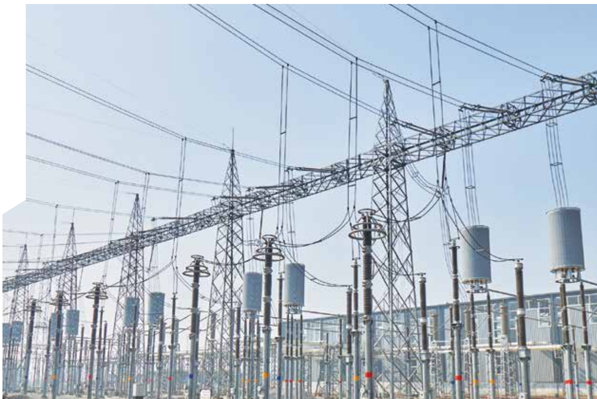
400kV Air Insulated Substation at Rajasthan
