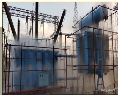
Commissioned 400kV 125 MVAR Bus Reactor for NTPC at Kahalgaon
