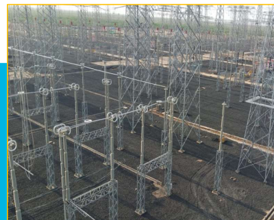
Commissioned 400 kV 03 bays & 220 kV 06 AIS bays for PGCIL at Bhuj
