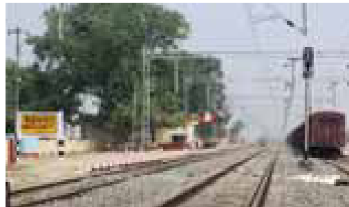
Mansi-Madhepura: Electrification Project
