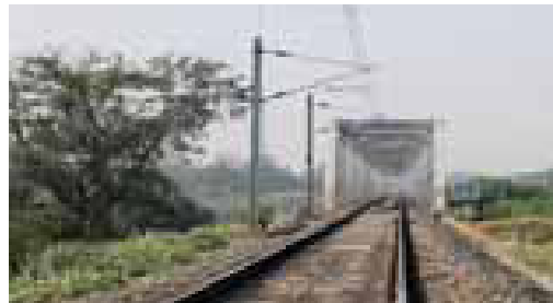
Chupra-Allahabad: Electrification and Signalling Project
