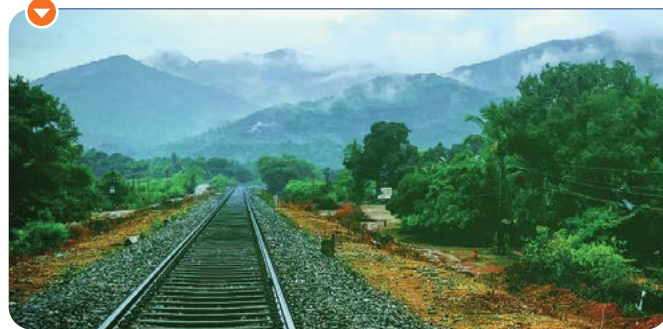
Verna Thokur Railway Project: Konkan region
