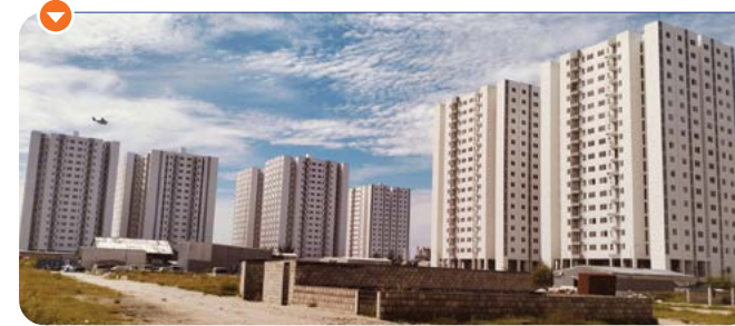
Social Housing Project, Maldives
