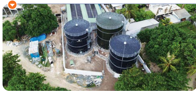
Construction of water and sewerage facilities including RTP and Admin buildings across 10 Maldivian islands.
