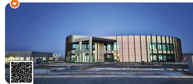
Mongolia Refinery Project located in Altanshree Soum of Dornogovi Province
