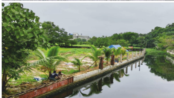
Development work started in Florence Grove, Kochi on the land beyond Thodu
