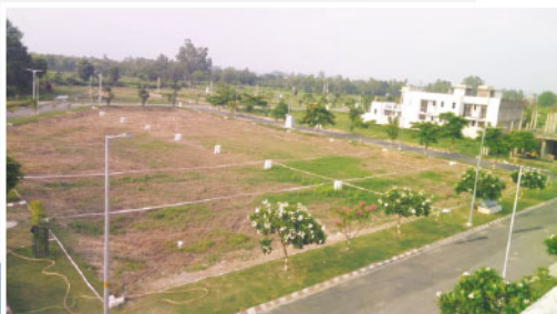
Aerial view of development work at Florence City, Pathankot.
