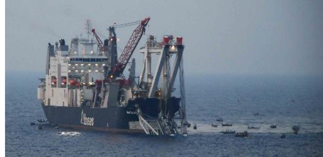
Deepwater Pipeline Installation Vessel: Audacia
