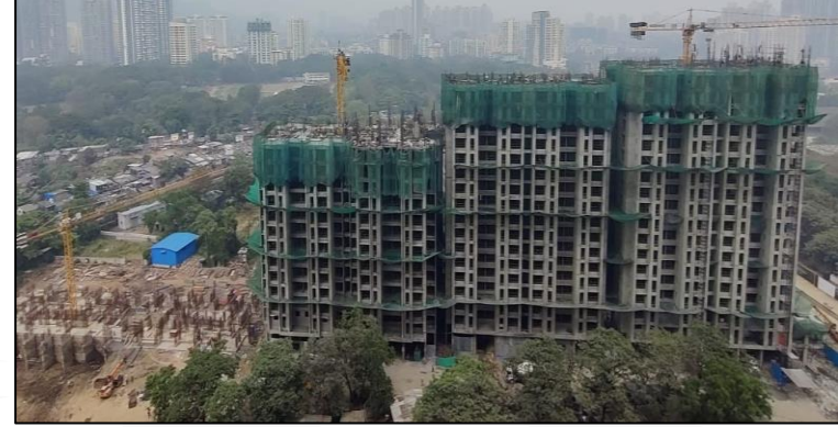
Tower No 6 -10 – Current picture
