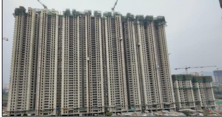
Tower No 1 - 5 – Current picture
