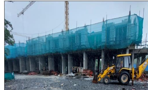
TOWER - 6 : 2nd slab WIP
