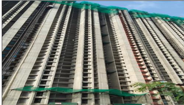
TOWER - 2 : 42nd slab ready to cast
