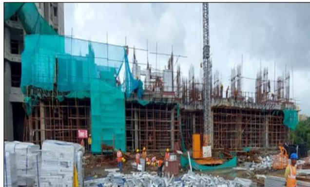
TOWER - 5 : 2nd slab WIP
