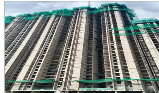
TOWER - 3 : 42nd slab ready to cast
