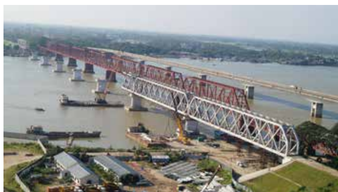
Superstructure Construction - Bhairab Railway Bridge, Bangladesh
