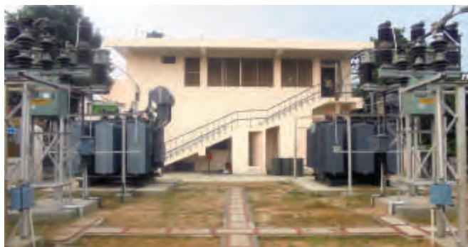
2x5MVA, 33 KV Sub-Station Jagriti Vihar, Meerut
