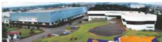
Menon Bearings plant at Kolhapur,
